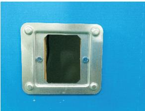
Using the anchors and screws provided for sheetrock or other suitable anchors, mount the monitor holding bracket to the wall. Tighten all 4 corners to the wall and make sure the back of the bracket is flush against the wall.
