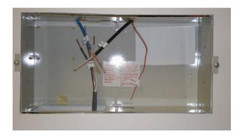
With the master removed, the housing should look something like this with all the wires disconnected and marked.
