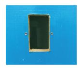
Cut a rectangular hole in the wall for the mounting bracket as shown. The hole should be approximately 2 inches by 2.3 inches.
